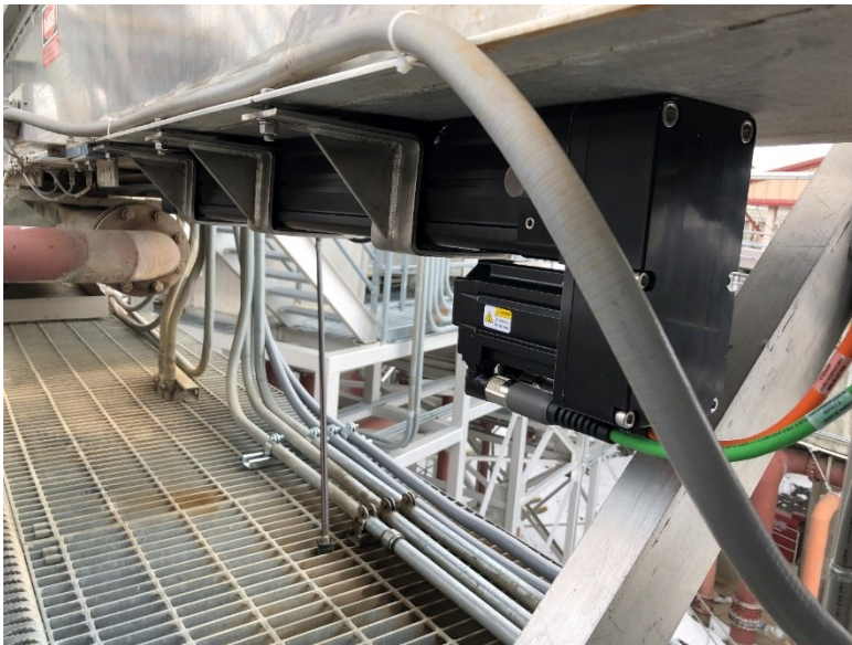
Figure 9. New electric cylinder at LJM A-B side gate.
