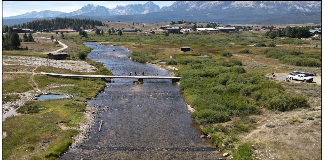
Figure 13. Aerial view of new PIT tag antennas on opposite sides of the bridge.
