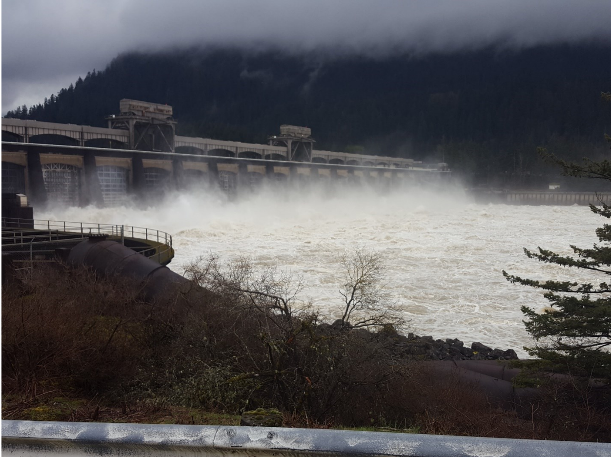
Figure 8. Bonneville Dam Powerhouse 1.
