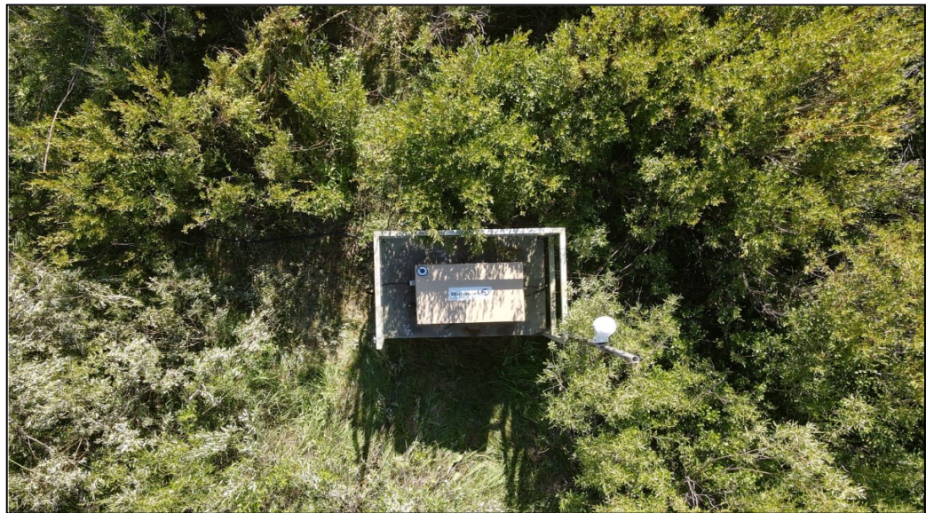
Figure 14. Aerial view of IS1001 MTS Enclosure.
